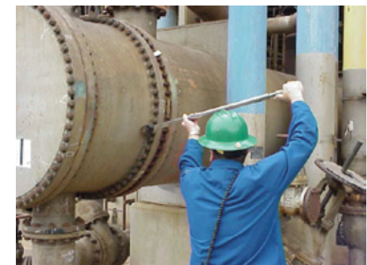
Traditional torque method
